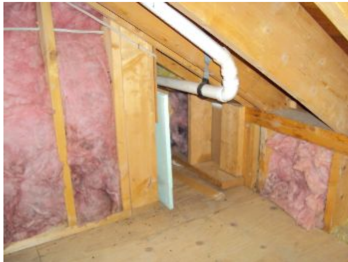
Attic Vent(s) Piping Through Attic
